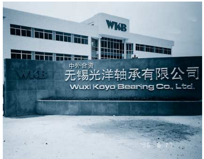
WUXI KOYO BEARING CO., LTD. (Wuxi, China)
